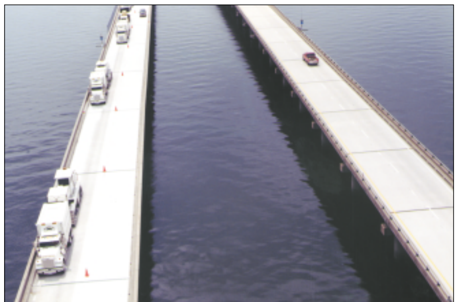
The texturing process for the Lake Pontchartrain Bridge in New Orleans took 25 days.
