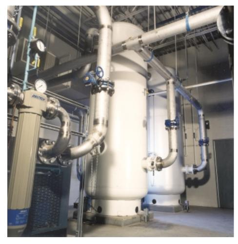
While orbital welding is frequently used in the semiconductor and pharmaceutical industries, this represents one of the first times it was used in construction of a water treatment plant. The use of this automated method increased productivity from 3 to 4 welds per day to 13 to 16 on the 6" to 8" pipe used for air distribution to the microfiltration system.
