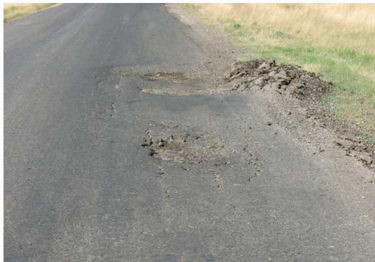
Left and above: Rural roads throughout Texas, like these pictured from the Laredo District, are deteriorating at a rate that has had alarming effects on roadway safety and economic development.
