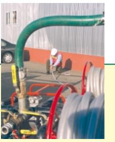
More than one hundred injection points were installed at accessible areas throughout the site and within the facility. About 150 gallons of remediation mixture was injected into each of the injection points during each of the three injection events. Average concentrations of both hexavalent chromium and TCE in the injection wells have been reduced 99.9 percent, and two on-site groundwater monitoring wells are not detecting hexavalent chromium.
