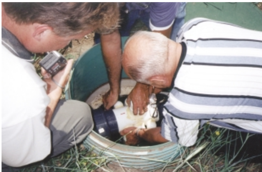
▲ The ultraviolet disinfection unit that receives effluent from a geotextile filter serving a development on Lake of the Ozarks is examined.
