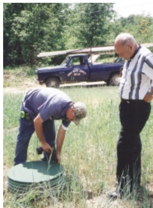
▶ George J. Gering, director of Public Water Supply District 2, adjusts the recirculating sand filter valve for a new cluster system serving 39 homes in Rolla, Mo.
