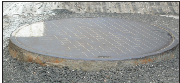
When left exposed like this, manholes can damage tires, rims, and undercarriages.
