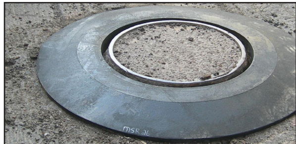
A raised manhole rim protected by a reusable rubber safety ramp—safe, convenient, cost-effective
