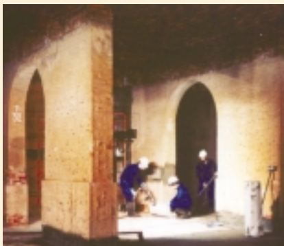
▲ After scouring the support to uncover a sound structural surface, a primer is applied that mineralizes the capillaries and microfissures, thus regaining cohesion in depth.
