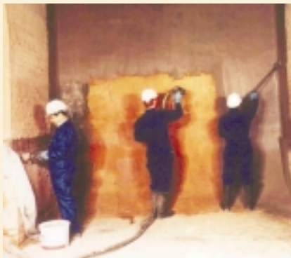
▼ Three layers of waterproofing product are sprayed on, the second layer being reinforced with a nonwoven geotextile.
