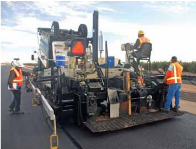
Research studies have shown that smooth asphalt pavements are a “win-win.” The asphalt contractors who built the award-winning roads in this story share one thing in common: They all used an electronic grade-control system to control the screeds on their pavers.
