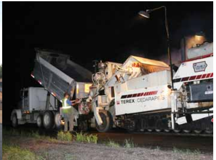
Research studies have shown that smooth asphalt pavements are a “win-win.” The asphalt contractors who built the award-winning roads in this story share one thing in common: They all used an electronic grade-control system to control the screeds on their pavers.
