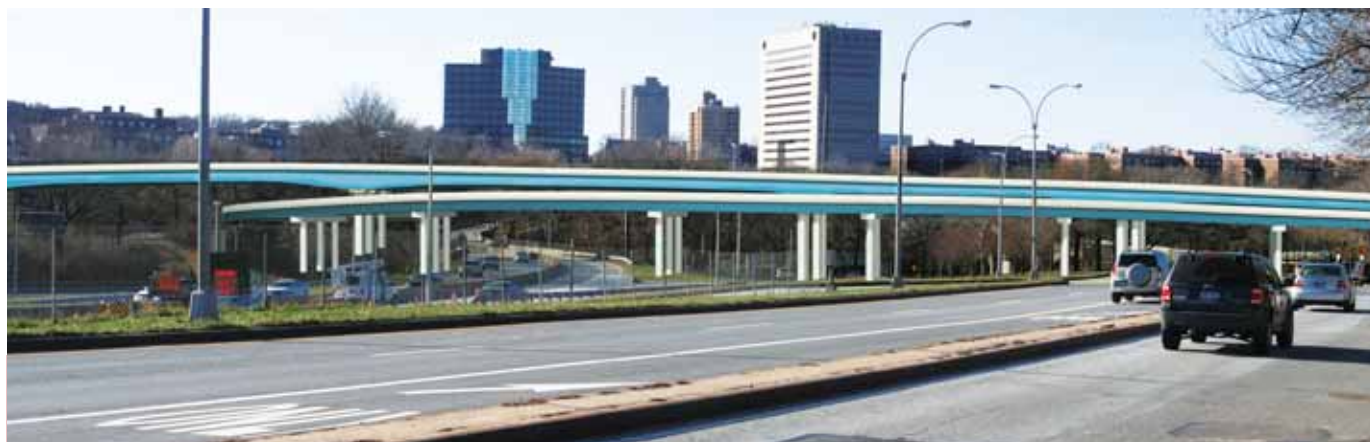
The proposed viaduct will be a four-span, continuous, steel-plate girder, with span lengths of 192 ft, 213 ft, 213 ft and 179 ft for an overall length of approximately 800 ft. The vertical profile has a crest curve along with horizontal compound curvature.
