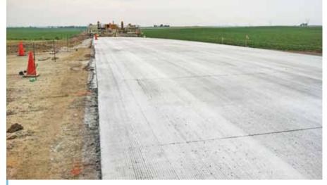
The flexibility of using PCC as a construction material has been much improved in lowa through the use of the maturity method. Better admixtures also have allowed crews to transport mix over greater distances and with larger placement windows.
