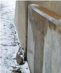
For both new construction and structural rehabilitation, requiring epoxy-coated or other corrosion-resistant reinforcement across the footing interface, coupled with waterproofing the interface, represents the current best practice for mitigating potential deterioration of J-bars or dowel bars near pier/stem wall-footing interfaces.
