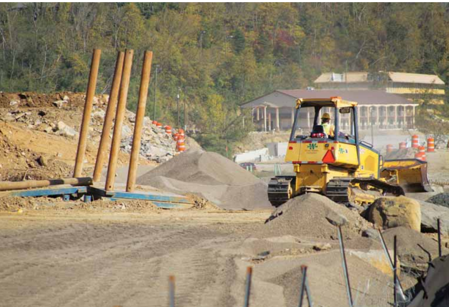
An average of 10 trucks a day delivered loads of lightweight aggregate from the Livingston facility, about two hours south of the jobsite. Because it is lightweight, coarse and noncompacting, a straight mix could be used to backfill the trench, directly on top of the culvert.
