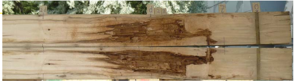
Figure 2. Wave speed vs. position on a laterally separated, decayed post.
