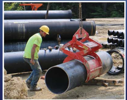
W.D. WRIGHT IS USING A PIPE LIFT™ TO SET 24 INCH DUCTILE IRON PIPE
