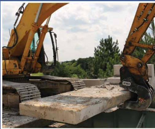
RIETSCHILIN CONSTRUCTION IS REMOVING THIS BRIDGE DECK WITH A SLAB CRAB®
