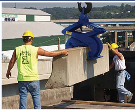
BRAYMAN CONSTRUCTION USES A BARRIER LIFT TO MOVE PRECAST CONCRETE WALL
