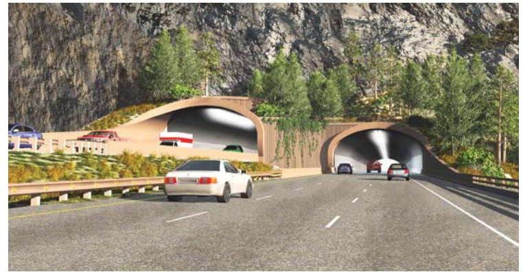
The new "Twins" offer three 12-ft driving lanes, a 4-ft inside shoulder and a 10-ft outside shoulder, as well as portal extensions beyond the rock face.
