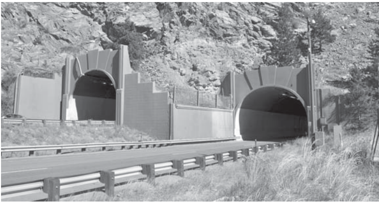
The original Twin Tunnels on the I-70 Mountain Corridor were completed in 1961. The tunnel portals were never subsequently augmented to prevent falling rock or debris from reaching the roadway.
