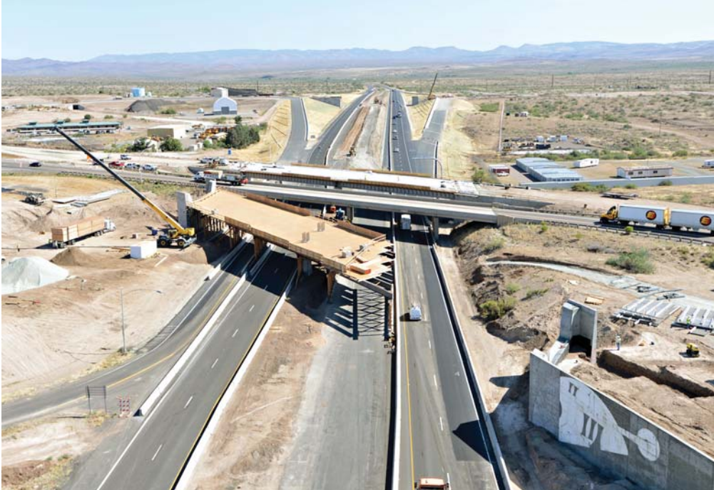
In order to keep traffic flowing during the reconstruction of the Cordes Junction Traffic Interchange in Arizona, Sundt and its joint-venture partner constructed one of the bridges over live interstate traffic. The photo shows the falsework that was created to safely perform that portion of the project.
