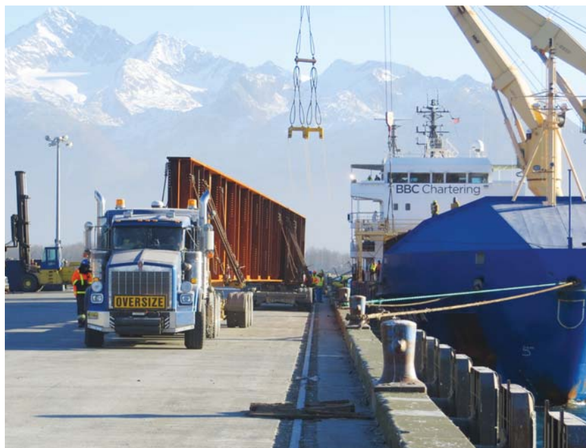
One of the major challenges of this project involved transporting by truck 80 165-ft-long girders 330 miles on the Richardson Highway from the port of Valdez, Alaska, to Salcha, Alaska. The girders were fabricated in China and shipped to Alaska.
