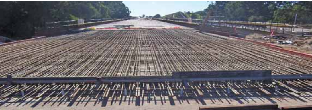
A closure-pour sequence, which relies on the closure-gap reinforcement resisting compressive forces as well as tensile forces, was developed in Australia.
