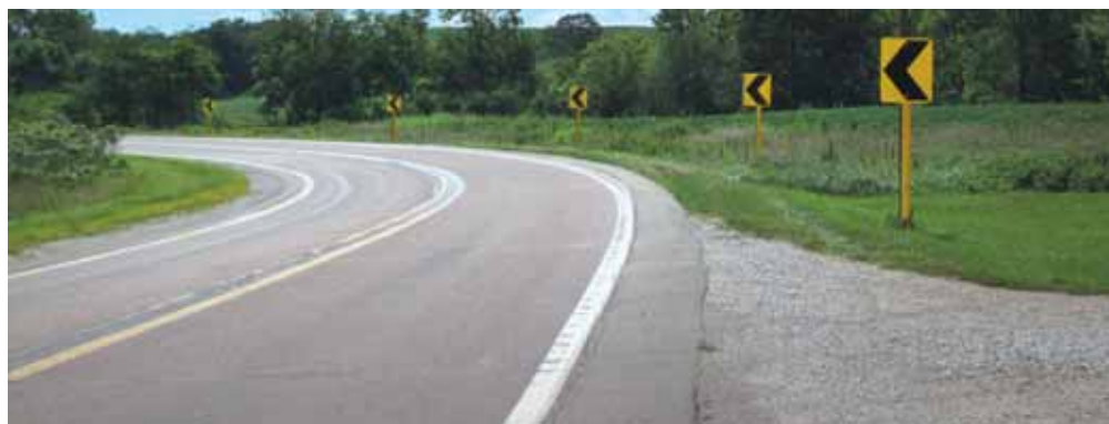
Reflective post treatments were added to the posts of existing chevrons at four curves. The post treatment adds delineation to reinforce the presence of a curve to drivers.
