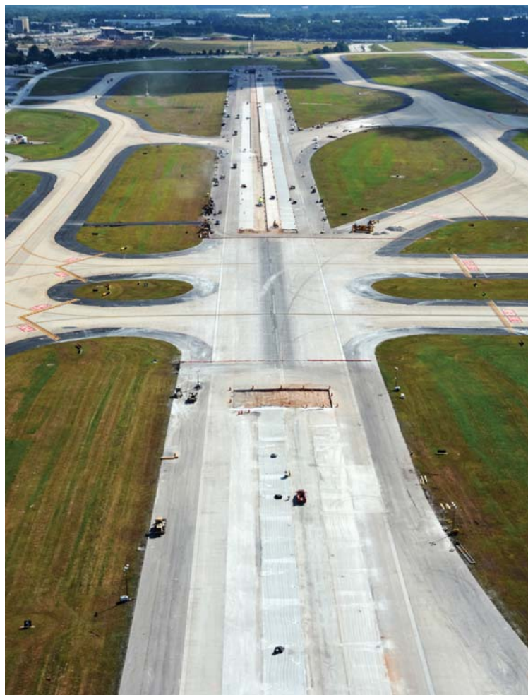
When all was said and done, the 8L/26R project employed 60,000 cu yd of concrete and required more than 210,000 man-hours over just 29 days.
