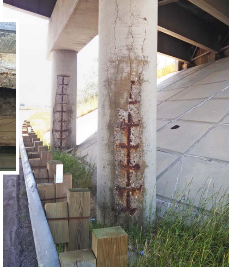
While concrete road and bridge structures are designed for a lifespan of 50-75 years, many do not make it even half as long, mostly due to degradation from within caused by pervasive corrosion of steel reinforcement.
