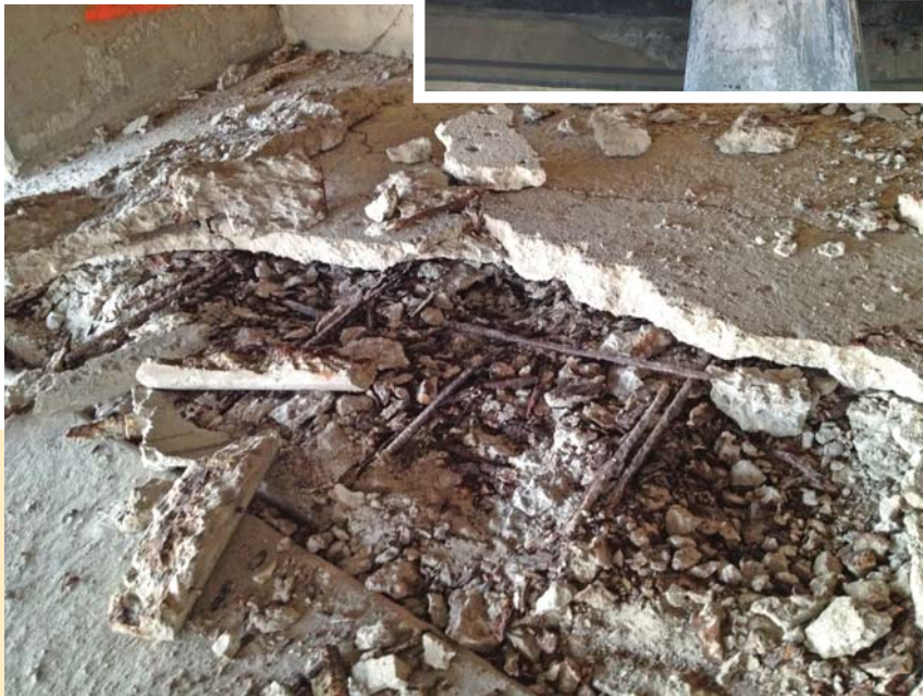
While concrete road and bridge structures are designed for a lifespan of 50-75 years, many do not make it even half as long, mostly due to degradation from within caused by pervasive corrosion of steel reinforcement.
