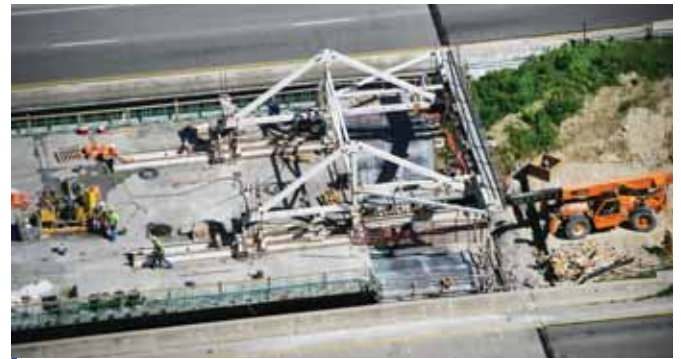
The cast-in-place construction process involves workers fabricating post-tensioned, reinforced concrete segments, 16 ft at a time. Because of the repetitive nature of this process, workers are less likely to make mistakes that will add to project cost.
