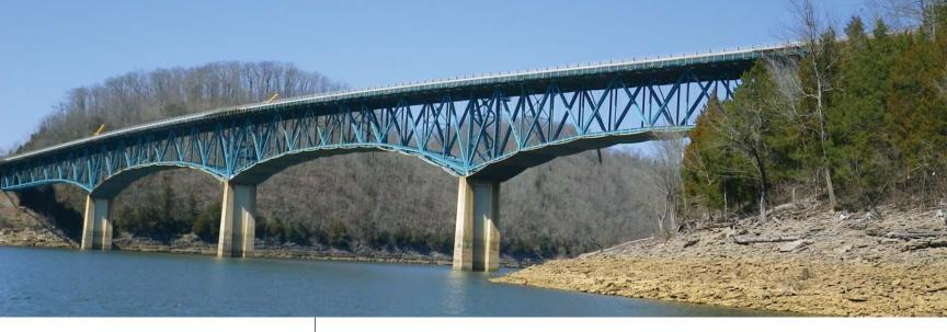
The continuous-truss construction necessitated very specific construction staging load patterns and intensities in order to prevent unacceptable stress reversal and to limit the magnitude of temporary stresses and loads on truss members and gusset plates. salts. This innovative design application should help increase the service life of the new deck and minimize future maintenance of the superstructure.
