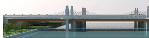
bridge. In addition, the project team used a steel trapezoidal box section for the edge girders, rather than a steel-plate I-girder section more commonly used on composite cable-stayed bridges. This was done to provide greater superstructure stiffness and less reliance on the cable stays, common on extradosed bridges. The project team also wanted to visually match the new mainline bridges (the current bridges are scheduled to be replaced with steel box-girder bridges).
