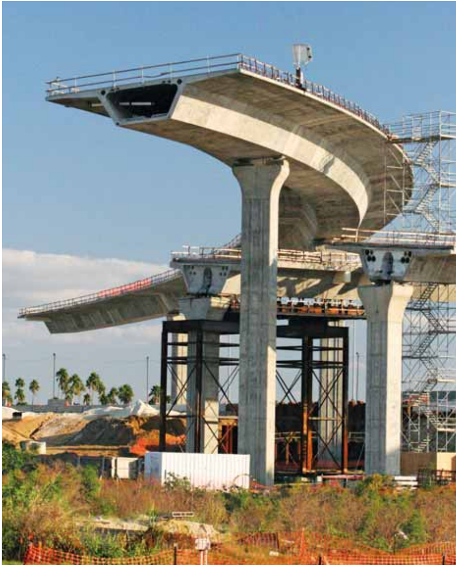
Accommodating roadway curvature for balanced-cantilever construction required the use of counterweights to balance the transverse loads induced by the curved superstructure.
