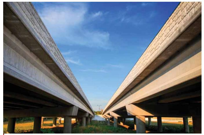
Estimated at \$23 million, the Stonebrook Parkway project, located in Frisco, Texas, includes a 3,800-linear-ft, six-lane major thoroughfare, twin bridges over a creek, a temporary railroad shoofly and a 195-ft, four-span railroad bridge.
