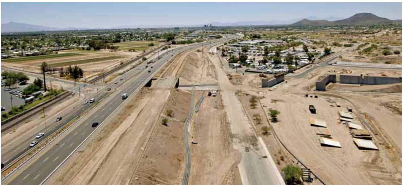
When complete, the Prince Road overpass will be 30 ft above ground level and will slope down on the east side of I-10 to reach ground level near Runway Drive. On the west side, the overpass will slope down and be realigned with a roadway called Business Center Drive.
