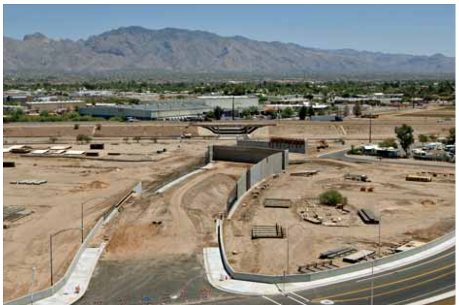
The improvements will allow traffic, including emergency-service vehicles, to pass over the railroad tracks without having to wait for the 40 to 60 trains that pass daily through the area and cause vehicles to back up onto I-10 during peak hours.
