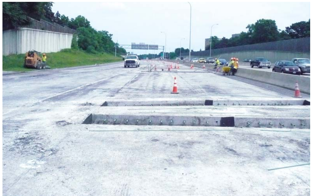
Compromised asphalt overlay was removed, allowing crews to address the underlying deficiencies in the concrete on I-394—in some areas performing a full-depth excision and repair.
