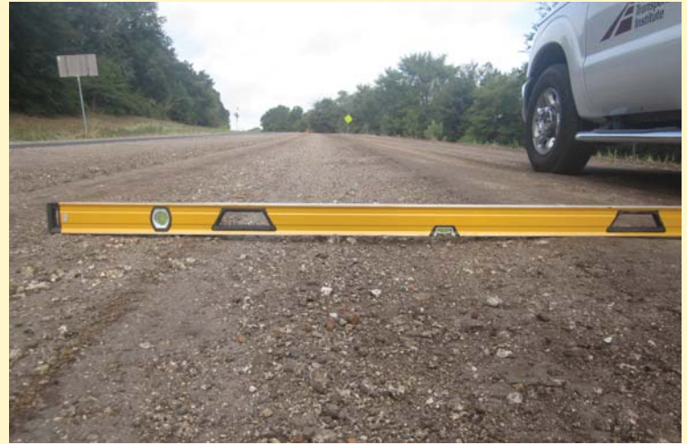
Figure 5. Failure under early traffic due to excessive compaction moisture content.
