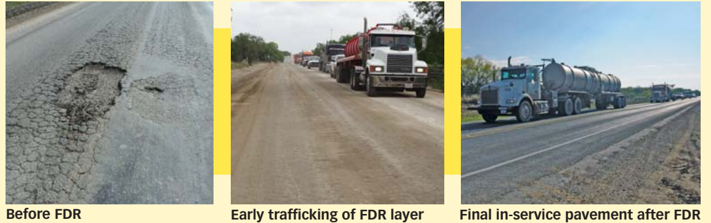
Figure 2. A successful FDR project was opened to energy-sector traffic within two hours after compaction.
