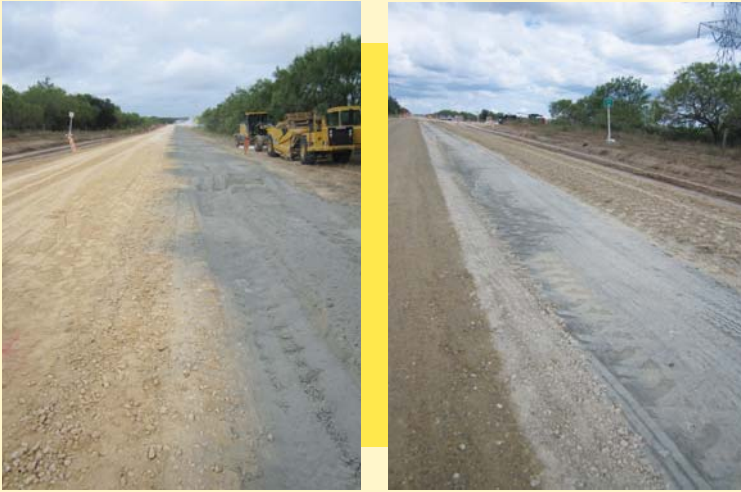
Figure 4. Contrast of uniform (left) and non-uniform (right) stabilizer application.
