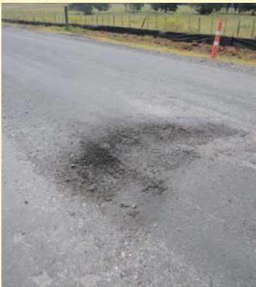
Figure 6. Local failure due to excessive water at location of disconnecting FDR train.
