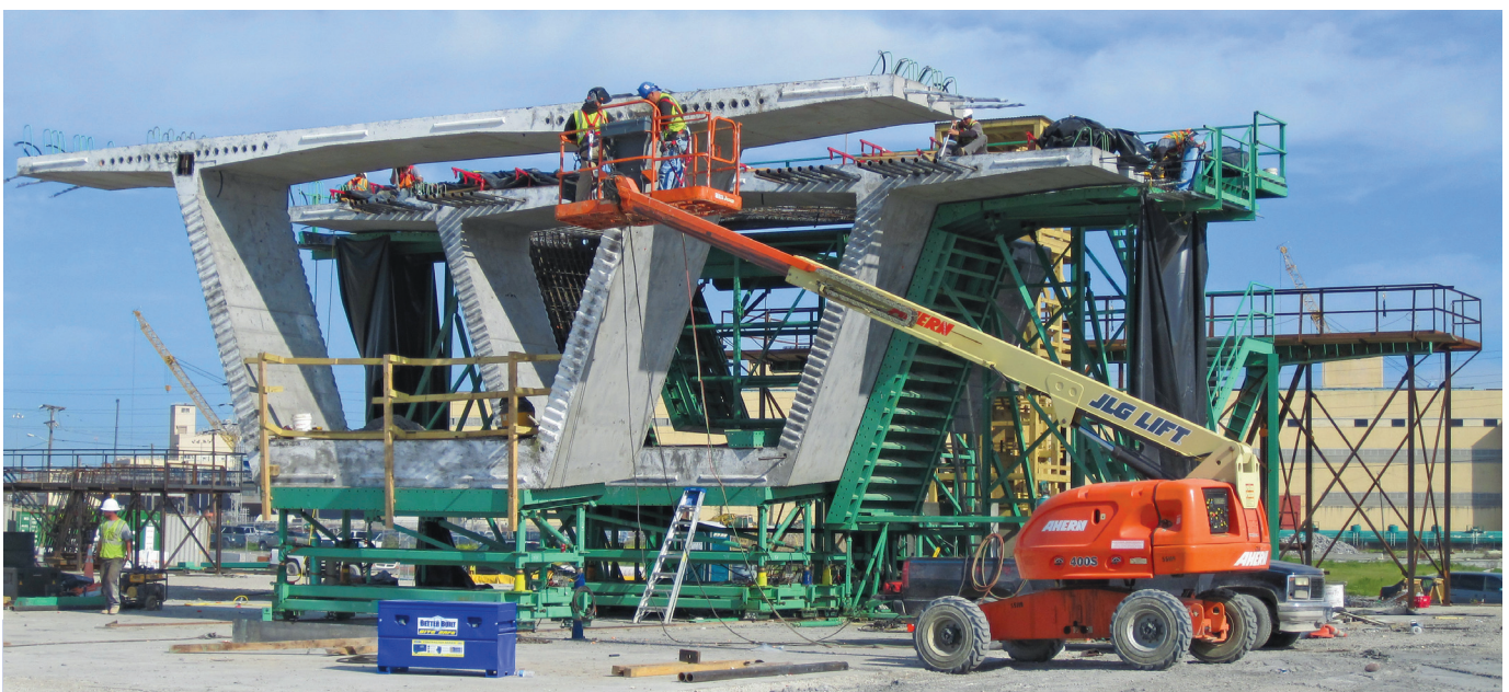
A total of eight precasting beds were set up in the casting yard: two for pier column segments, four for the typical-span superstructure segments and two for the variable-depth main-span superstructure segments.
