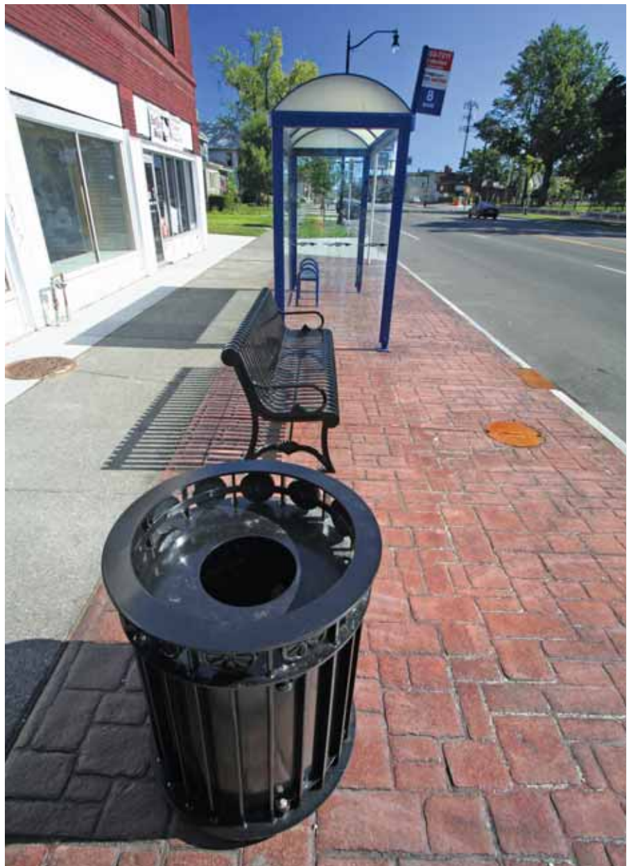
All sidewalks of the project were replaced using an exposed aggregate mix, which lends a historic texture to walkways. Snow-storage strips were replaced with red-tinted concrete with a block stone pattern and gray release.
