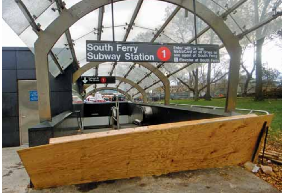
All eight subway tunnels, major stations and rail yards were flooded in the worst storm damage in the MTA's history. By Nov. 3, 80% of the subway system was in operation.
