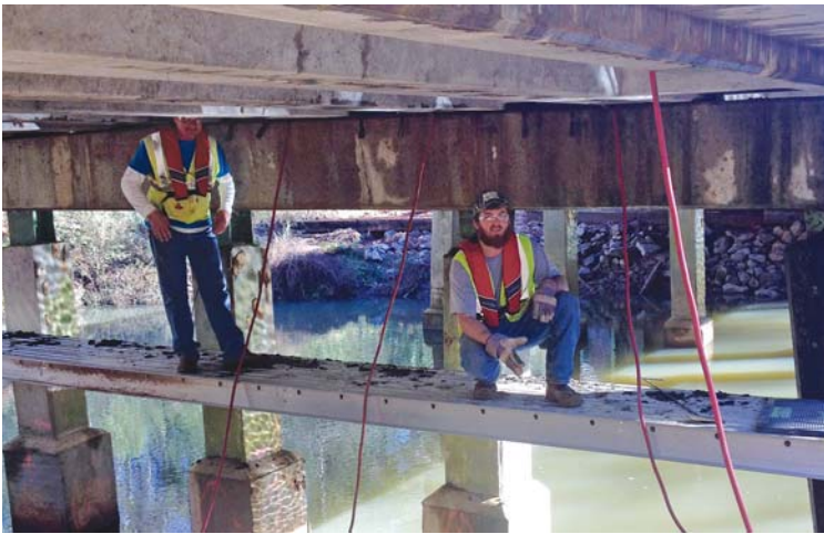
The timeframe for the bridge bearing-pad-replacement repairs ranged from 3-5 days from setup to completion depending on the length of the bridge.
