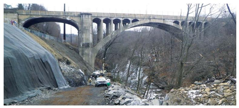
A condtion survey concluded that the upper portions of the bridge, including the deck beams, deck arches and deck itself required complete replacement.
