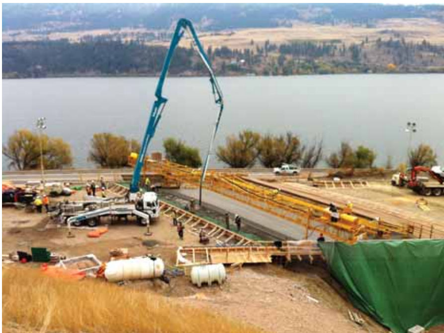
The contractor set a paving productivity goal of 880 to 1,060 cu ft per hour. Within 4.5 hours, the crew put the finishing touches on the bridge deck.
