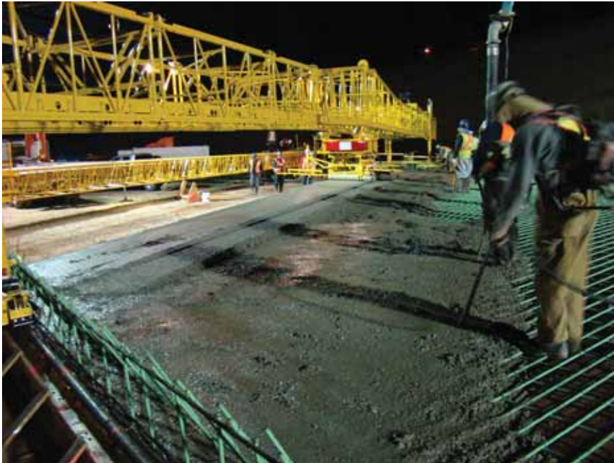
Increasing the complexity of the pour, the deck had a 5% grade, so from previous experience Camwood crews had cable turfers ready to assist.
