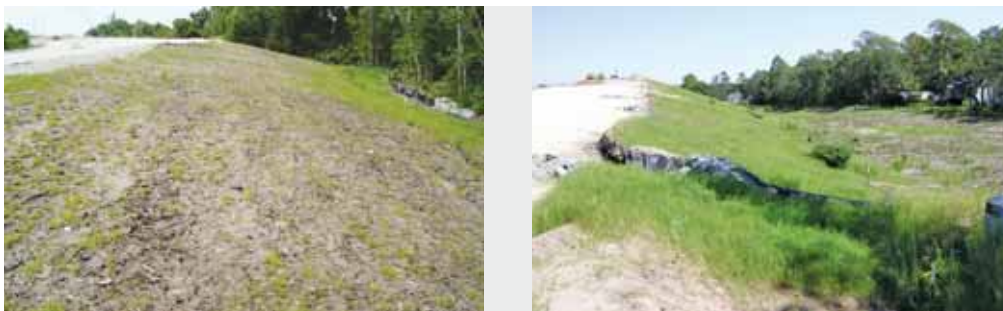
Figure 3. Compost seeding initial application with germination (left); dense vegetative coverage (right).
