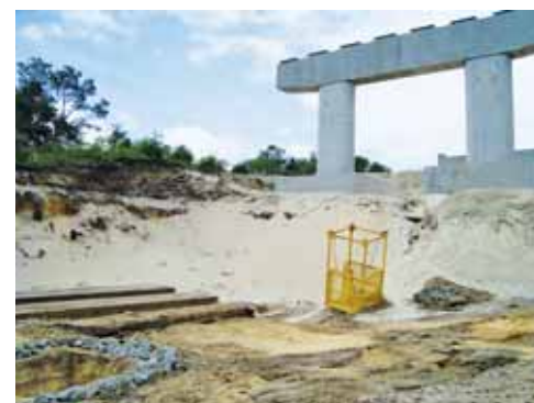
Figure 1. Fine sandy granular soils encountered on a barrier island bridge project.
