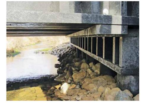
The abutment backwalls of the Onion Ditch Bridge are 3-in. x 12-in. planks screwed into pilings that were driven in a line 3.25 ft on center at each abutment. Bridge seats at both abutments are 18-in. structural plastic I-beams.
