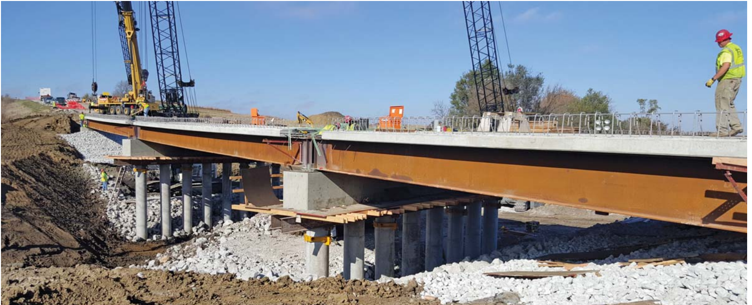
Crews working on one of the three spans of the Little Silver Creek Bridge in Pottawattamie, Iowa.
