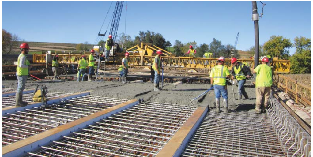
A concrete pour is being performed for deck pre-fabrication.
