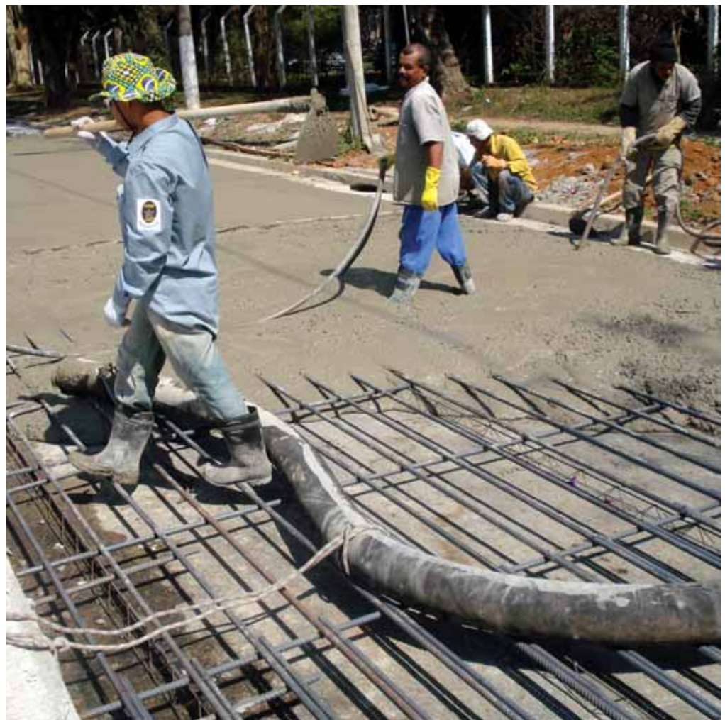
The first continuously reinforced concrete pavement in Brazil was built at the University of São Paulo during the winter of 2010. It was originally intended to verify, for tropical conditions, the occurrence of transverse cracks and its comparison to crack patterns in other climates.
