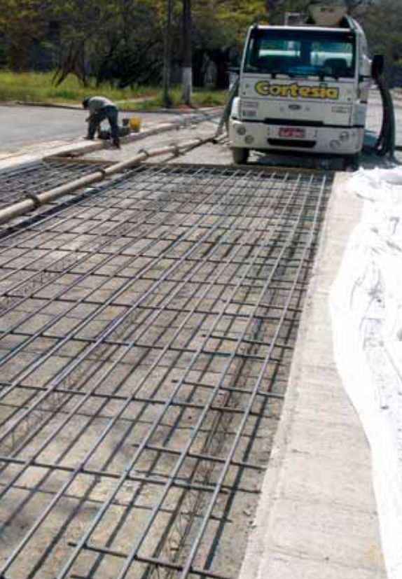
The short CRCP sections built at the University of São Paulo developed a few transverse cracks since construction in 2010. After one year, the cracks were quite different from conventional CRCP.
