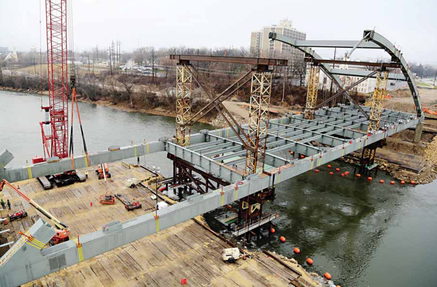
The Morgan Street Bridge/Corridor project includes a 503-ft, network tied-arch structure, along with roadway reconstruction projects on both sides of the bridge. Construction is scheduled for completion in December 2013. From the outset, a consensus emerged that this would be “more than a bridge.”
