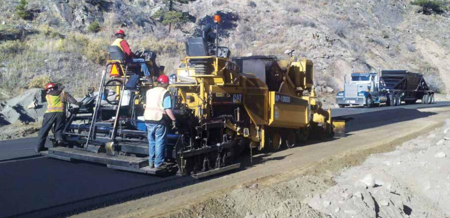
To maintain asphalt workability, forces of Coulson Excavating pave U.S. 34 between Loveland and Estes Park with warm-mix asphalt due to long hauls of up to three hours, low ambient temperatures at the end of the season and high elevations. Photo courtesy of MWV Evotherm.
