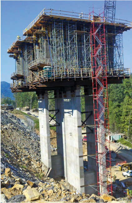
The main piers of the eastbound and westbound bridges are reinforced concrete columns. The vertical reinforcing steel is 75 ksi, surrounded by a low-permeability 5,000-psi-compressive-strength concrete. Each pier will use 300,000 lb of reinforcing steel.
