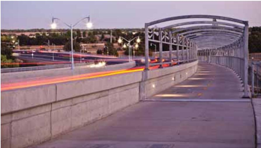
The steel wave pattern concept on the equestrian railing was added to soften the railing's appearance and tie in with the wave pattern on the outside precast girders. To limit the amount of excavation required for the construction of walls and footings, designers used different retaining wall types depending on location.
