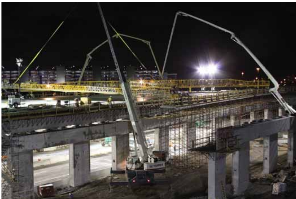
Runway paving was segmented into five different cells and the taxiway into six. Two pavers are being used to pave all four. Crews target a pour every three to four days.
