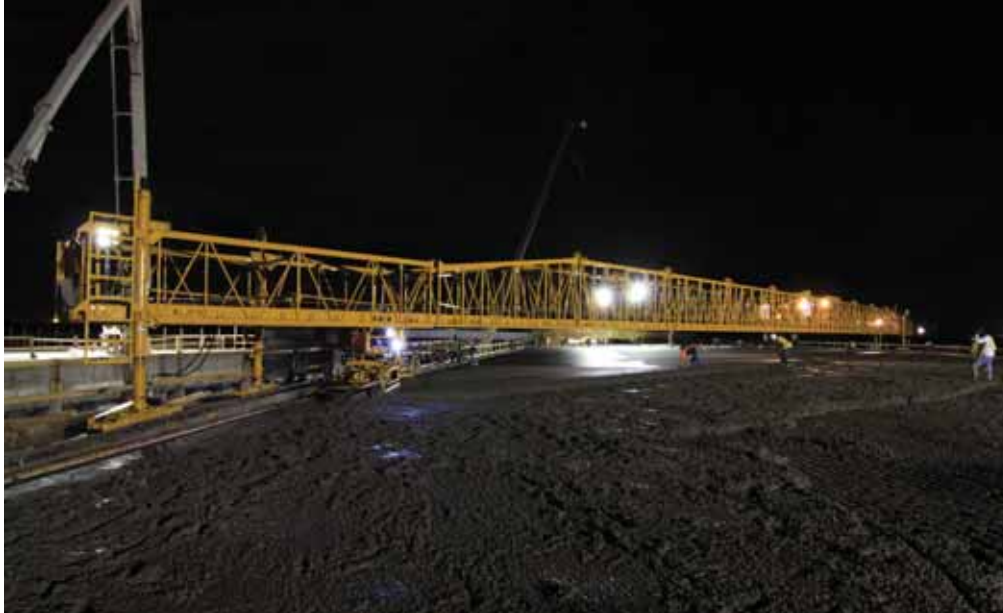
When paving at or over 180 ft, transition inserts are used to increase the paver's frame depth from 48 in. to 66 in., increasing frame rigidity and preventing deflection.
