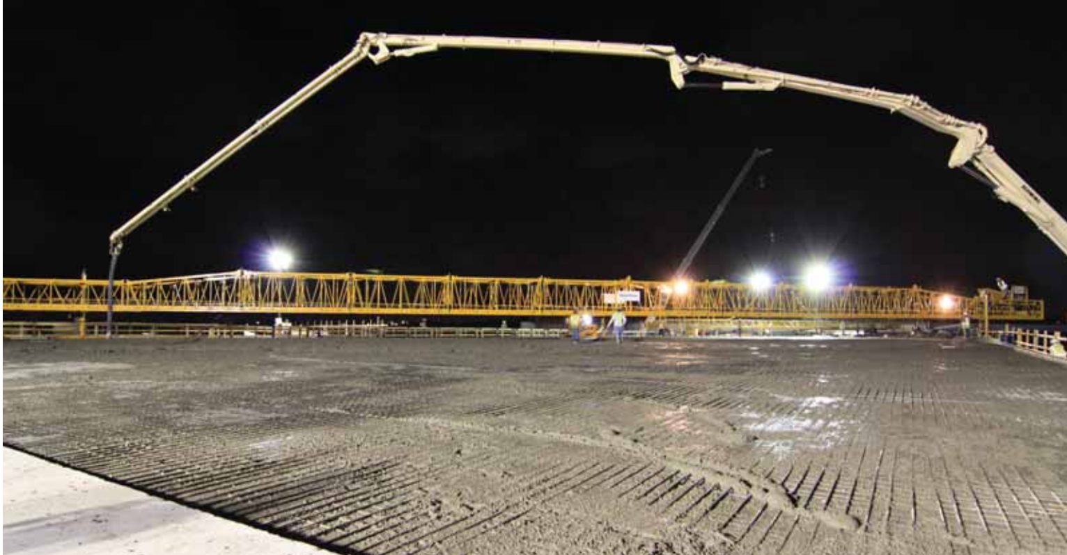
The first lift of concrete was loaded to the top mat of the rebar well in front of the paver to achieve proper beam deflection.
