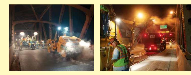
All work on the 1,000-ft twin-span three-lane bridge took place at night. Crews were allowed to close one lane at 7 p.m. and the second lane at 9 p.m. That left one lane open at all times. Sections of the road were milled and paved in a single night. Crews had to be off the road by 6 a.m. Bridge authorities were determined to make the resurfacing last.
