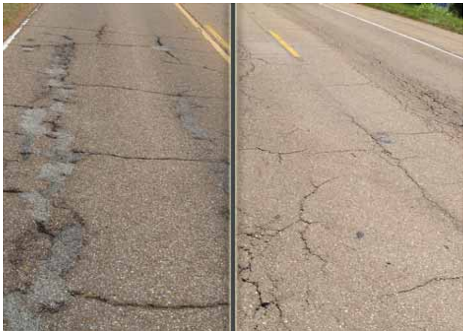
When performing reactive maintenance as a stop-gap measure on structurally unsound roads like these, the treatment life cycle may be greatly reduced.
