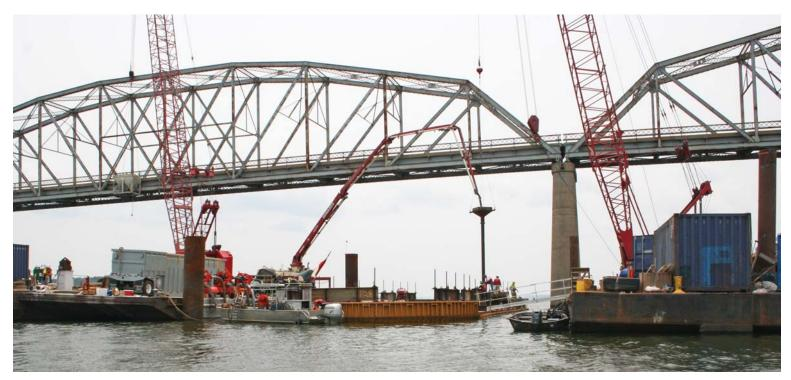
The shallow depth of the main span's tie girders will aid the navigation channel's improved vertical clearance.
