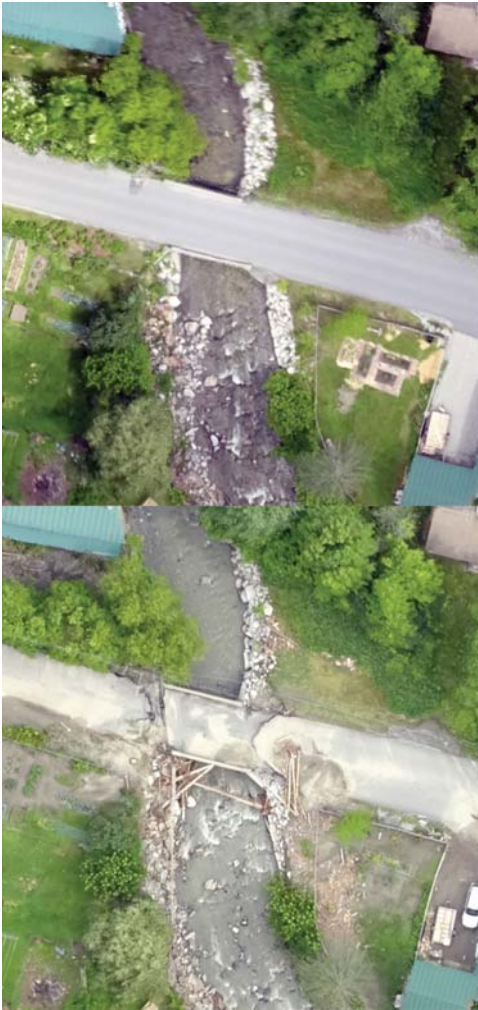
Figure 2. UAS assessment of bridge flood damage in Vermont earlier this summer.
