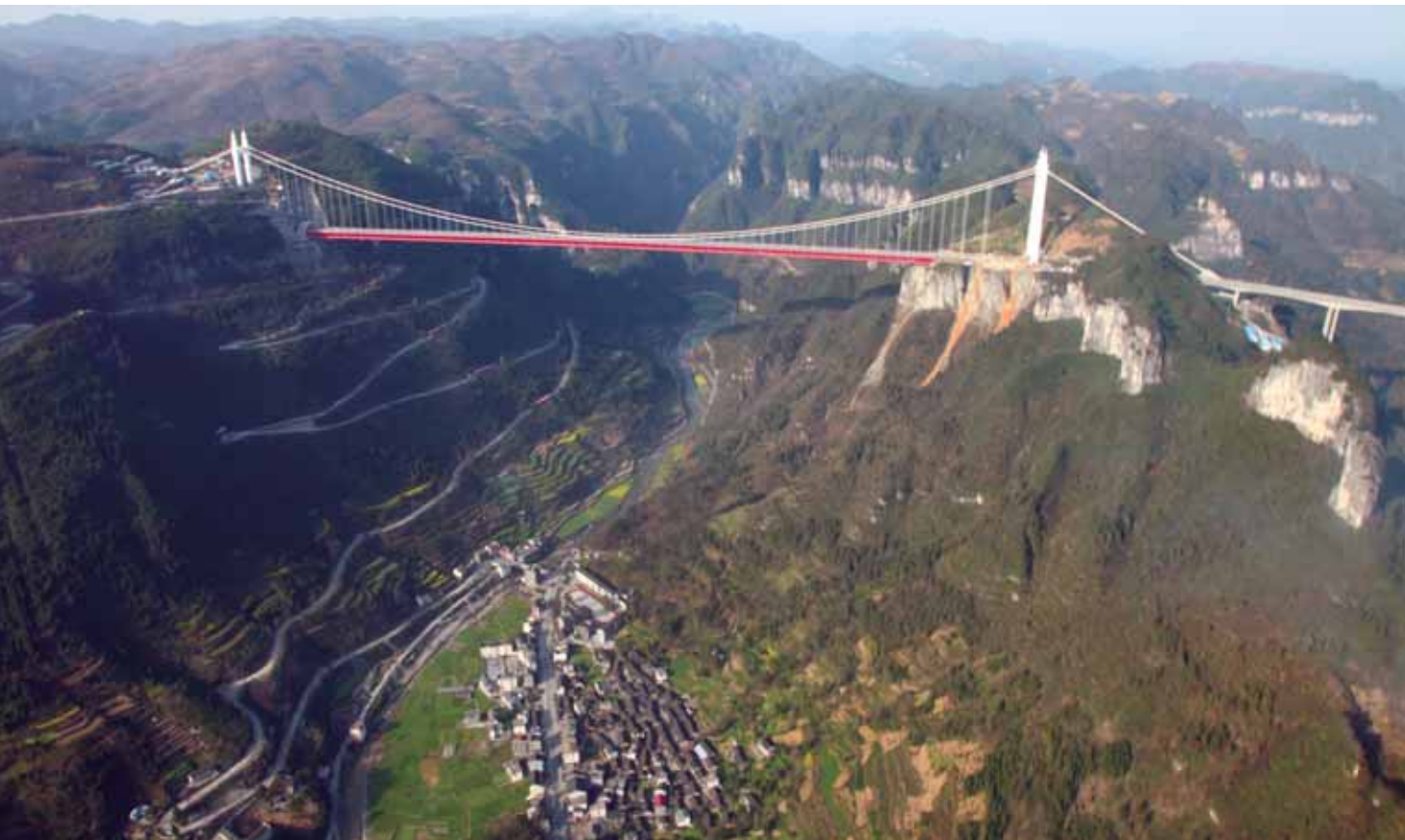
Since the Aizhai Suspension Bridge spans over a deep valley, the main span has to be directly connected to the tunnels at both ends. The direct connection presented challenges to both design and construction due to the requirement for the transition from the flexible bridge superstructure to the rigid tunnel structure.
