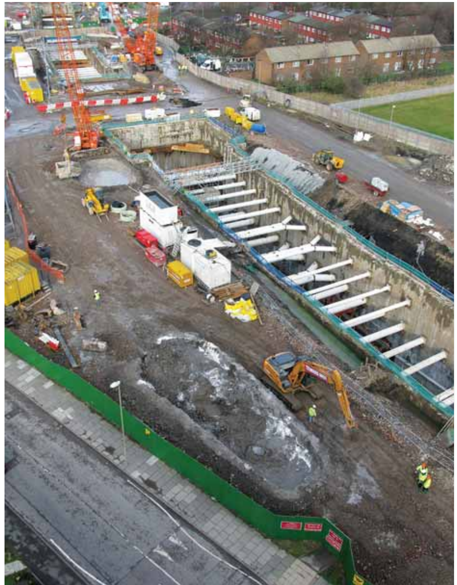
The northern approach will be 1,050 ft long and the southern approach will be more than twice that at 2,700 ft. The fact that the northern approach tunnel crosses over the existing tunnel with less than 10 ft of clearance presented one of the greatest challenges.
