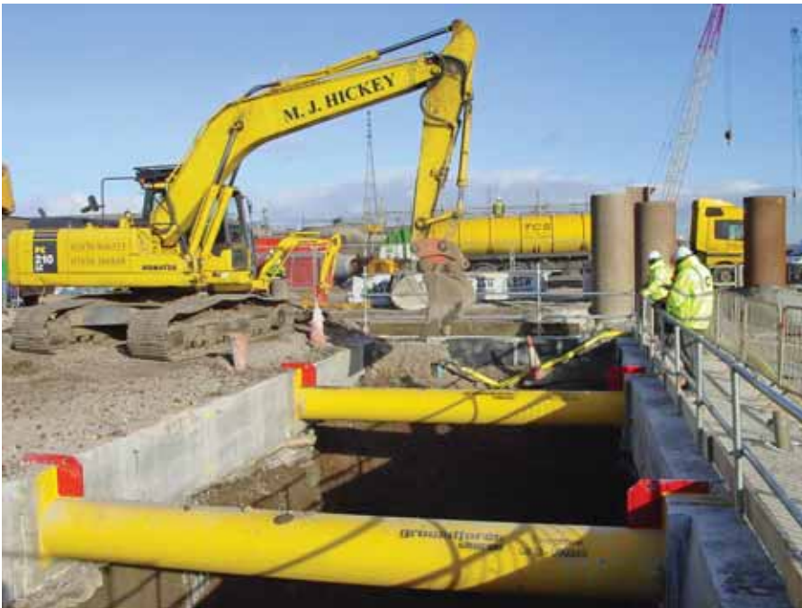
Workers excavate the tunnel area between the two diaphragm walls. Temporary props between the walls helped them withstand the high ground pressures.
