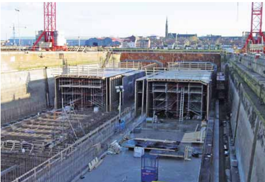
Scheduled for completion in December 2010, the $171 million project is being executed under a 30-year design-build-finance-operate-maintain concession.
